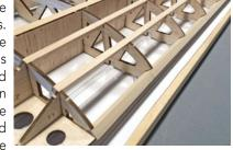
leading edge. Measure, cut and glue this in position. Be sure all three of these strips are glued to each rib.
